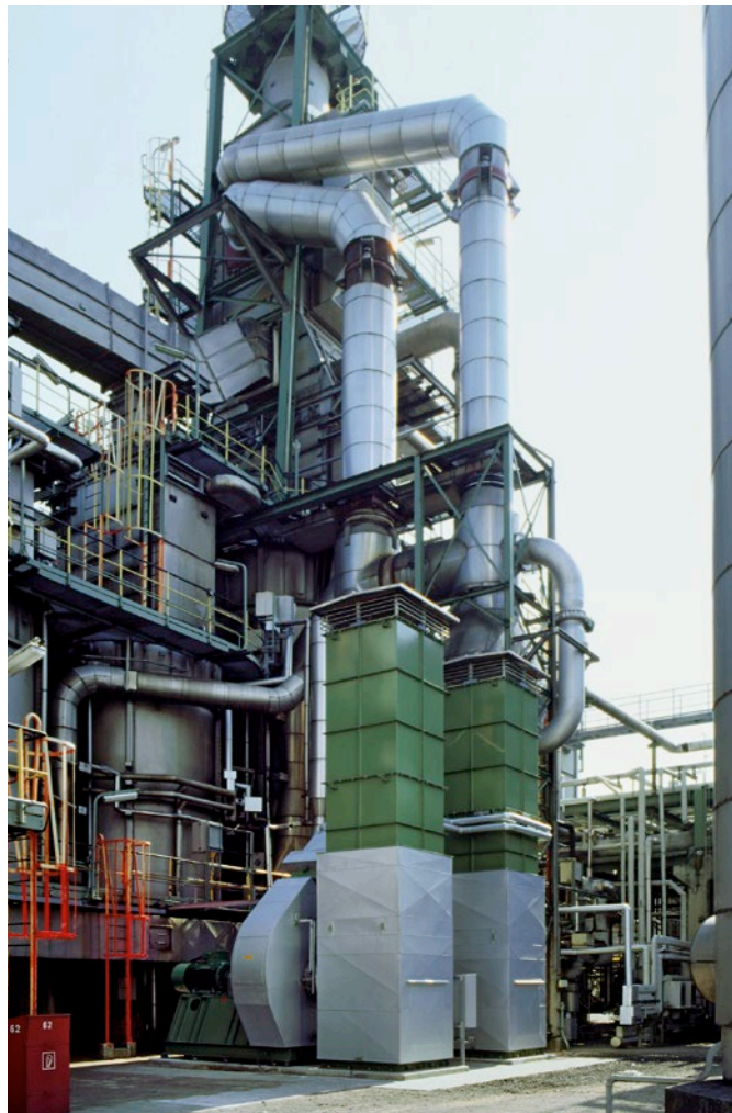
Fresh air fans in a refinery
