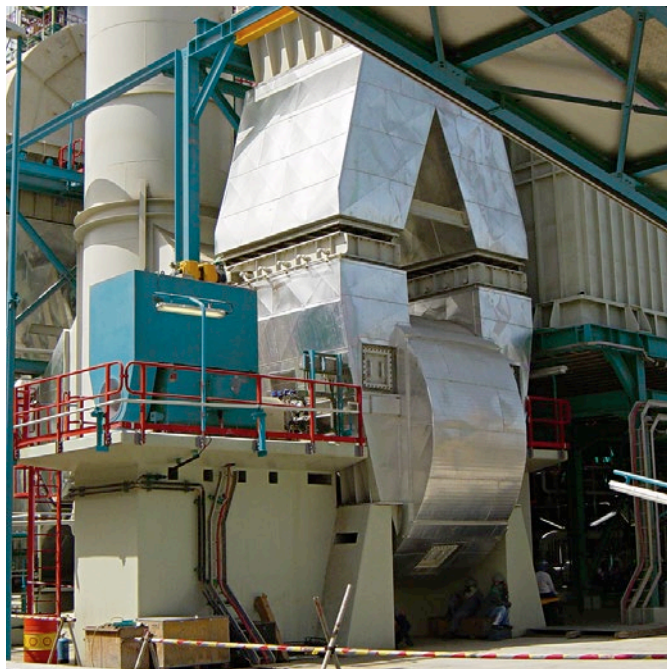
Exhaust fan behind wet scrubber for urea plant
